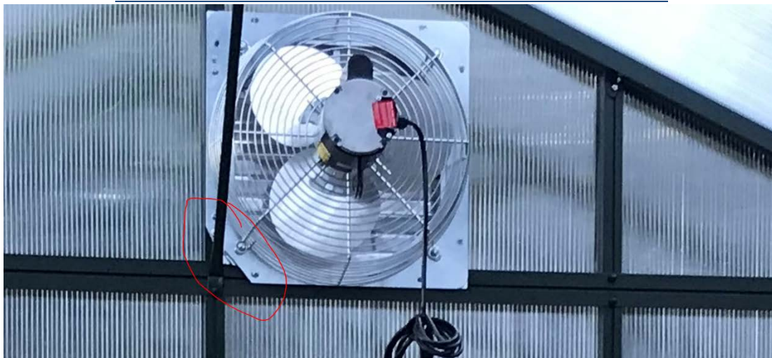
OPTION 1: Attach fan with bolts inserted into channel of PRO1456
