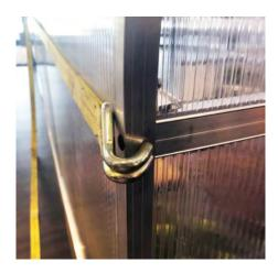
**Rubber Mallet:** start at the completed gable end and slide the polycarbonate panels as far as they can go into the channel. Then, hit the curved profile with rubber mallet. Hit the curve profile near the top and near the bottom to slide the profile evenly. It may help to have (2) people doing this. This will close the gap in the opposite gable end.
