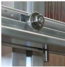
Insert one M6 x 12 bolt (S12) per greenhouse curve (including edge curves) into the lower bottom channel of the attached greenhouse lateral support.
