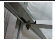
Attach the cross-braces (pos. 5) to the greenhouse lateral support with inserted bolt and nut and let them hang.
