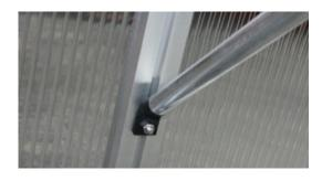
Attach strut to greenhouse curve with bolt (S5) and nut (S1). Tip: Insert bolt (S5) at the insertion point near the bottom of the curve. Please note that the black angle may not match the angle of your greenhouse curve.
