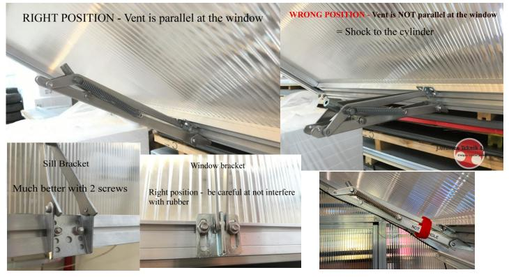
If you do not want your roof vents to open/close automatically during the wintertime, the red strap included with your kit may be used to hold the roof vents closed. This will prevent wind from blowing the roof vent open. You will have to disengage the piston entirely. If the piston is engaged with the red strap attached, the pressure will cause the piston to burst. Unthread the piston from the threaded circle collar to disengage the piston - you may leave the cotter pin in place.
