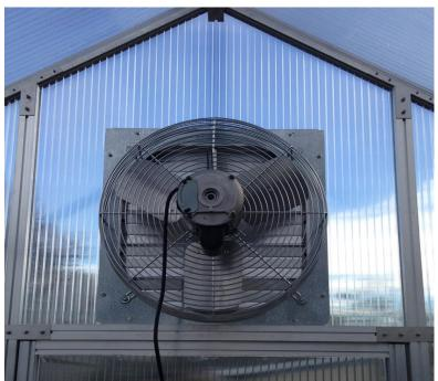
For the Riga XL the best placement is above the rear wall door with the weight on the door frame as seen to the left.
