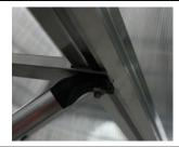
Attach crossbrace to front longitudinal profile (from shelf kit) with inserted bolt. Add the strut assembly beneath and tighten with nut. Repeat on all curves.
