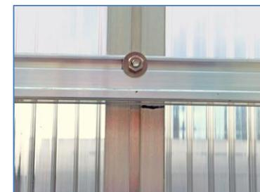
5. If you ordered an extra pair of lateral supports to use as hanging points, install them at any convenient height above the slanted T connectors, but be sure to keep them clear of the automatic window openers.
