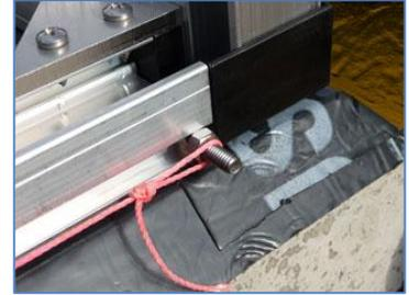
Make diagonal measurements as you square the floor profile rectangle. Accuracy is very important; always measure from and to identical points that are mirror images of each other. The profiles are ready to be anchored when the measurements are equal and all four string lines reveal no bowing.
