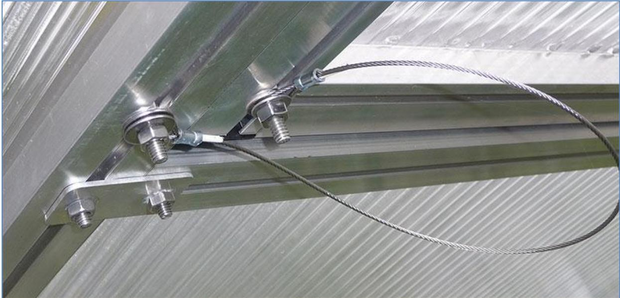
Two restraints are used for each window; one on each side. Install each loop between two flat washers on screws that were loaded in Steps 1 and 11. Position the restraint as illustrated and adjust as needed to avoid interference from the crossbar as the window is raised and lowered.
