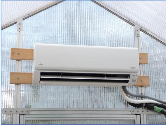
Ductless mini-split heat pump indoor unit
