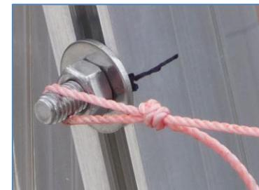
4. After making the marks remove the string and place a lateral in position, retained on each end by the screws in the gable arches. Install the remaining screws pulling the lateral away from each arch as needed to get it over the screw. The marks indicate the position of the lateral's bottom surface corner – if it had a corner. Since it is beveled, you must project where the corner would be as you fasten to the arches.
