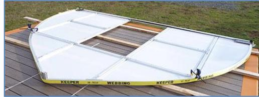
Pre-drill a clearance hole in each end of the floor profile for a #6 stainless self-tapping screw, ½ inch long. Drive the screws into the plastic corner connector to temporarily secure these parts against separation while moving the gable or tilting it into position. You might need to remove these screws later when you connect the side wall floor profiles.
