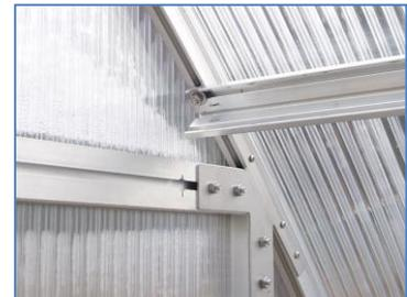
3. Locate the preloaded M6x16 screws at the marks and fasten the nuts tight. Stretch a gable-to-gable string between like screws and use it to make marks on each of the side wall arches. You may notice that the side wall arches are deformed inward by the force of the curved glazing; more so near the center than near the gables. Attach the string near the ends of the screws to minimize drag on the arches and provide a better straight line.
