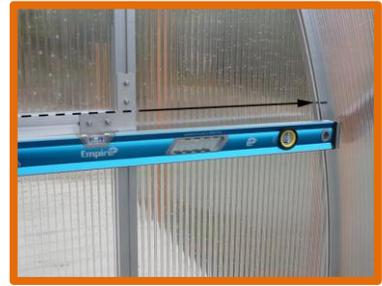
2. For the upper laterals, make a mark on the concave face of each gable arch at the end of the K connector's upper arm. This will be approximately 1968 millimeters above the substrate. This elevation is optimal for structural purposes but may not be best to support an optional upper shelf. If shelving is in your plan make the mark at your preferred shelving elevation. Instructions for shelf installation are [here](#).
