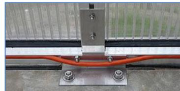
An ordinary 16 gauge extension cord fits nicely in the screw capture slots. Press it into the slots along its route to keep the walkways clear.
