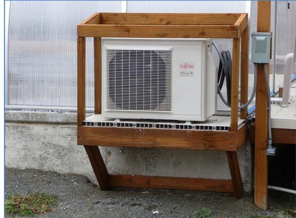
Ductless mini-split heat pump outdoor unit
