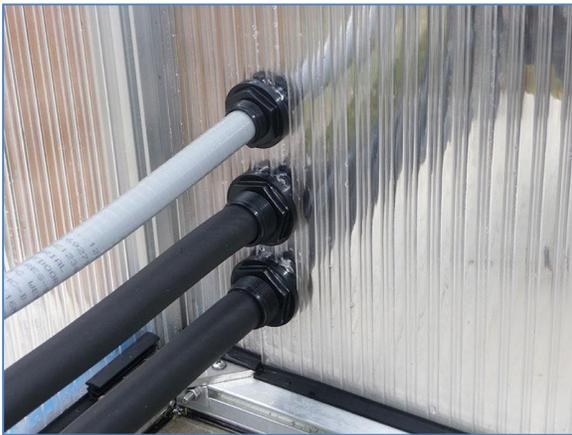
Glazing penetrations for refrigerant lines and power
