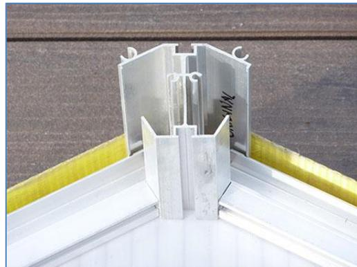
Clamp the corner junctions and confirm that they are square and properly positioned before driving self-drilling screws through the connector plates into the arches.
