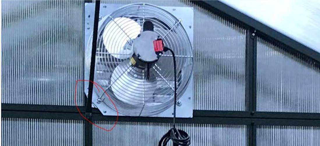
Once your panel with the cutout for the fan is in place, mount the fan on the interior of the greenhouse using bolts in the channels of the aluminum extrusions. These bolts will fit through the holes on the exhaust fan. You may need to cut the corner off due to the diagonal support beam being in the way. Once the fan is mounted on two sides to the aluminum extrusions caulk around the area where the box of the shutters meets the glazing.
