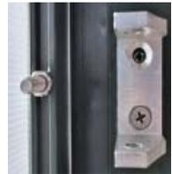
Next, hold the lower U-shaped mount up to the crossbar and mark the center of one hole. Using a 1/8" drill bit, drill the first hole, then screw the bracket on, check for level - then mark and drill the second hole. Slide the brass part of the opener over the bolt in the window channel. Use the supplied nylock nut to secure the opener on the top mounting bolt. Finally thread the large side bolts into the U-shaped mount and the opener is installed.
