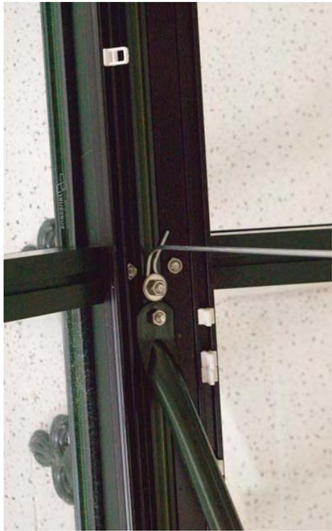
Note: If curtains are going to be installed, the misting system should be hung with bolts as shown to the left. The hangers will need top be bent into position.
