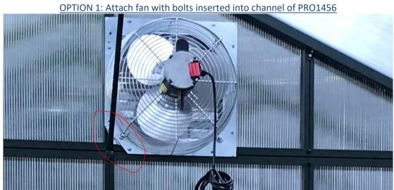
Once your panel with the cutout for the fan is in place, mount the fan on the interior of the greenhouse using bolts in the channels of the aluminum extrusions. These bolts will fit through the holes on the exhaust fan. You may need to cut the corner off due to the diagonal support beam being in the way.
