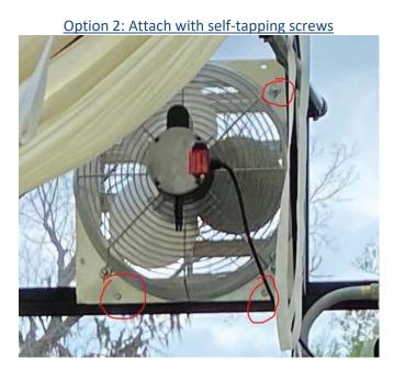
Conversely, you can use self-tapping screws to hold the Exhaust Fan in place. Pre-drill holes in the exhaust fan metal to match up with the Pro1456 Gable piece. You may need to cut the corner off due to the diagonal support beam being in the way. Once the fan is mounted on two sides to the aluminum extrusions caulk around the area where the box of the shutters meets the glazing.
